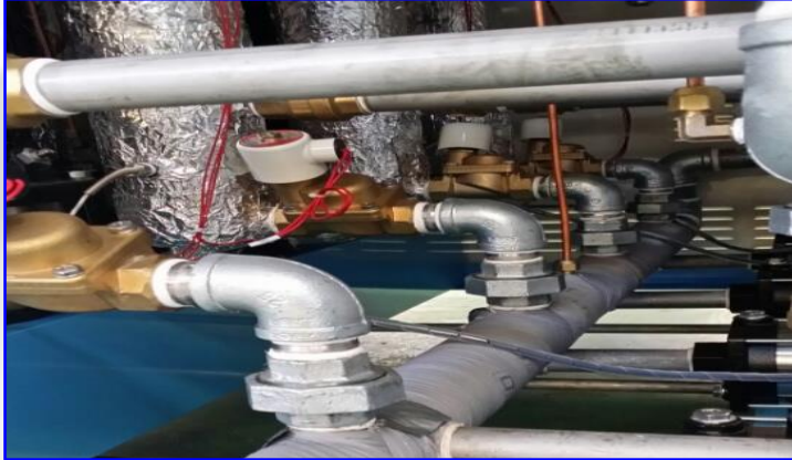
Platform / piping work
